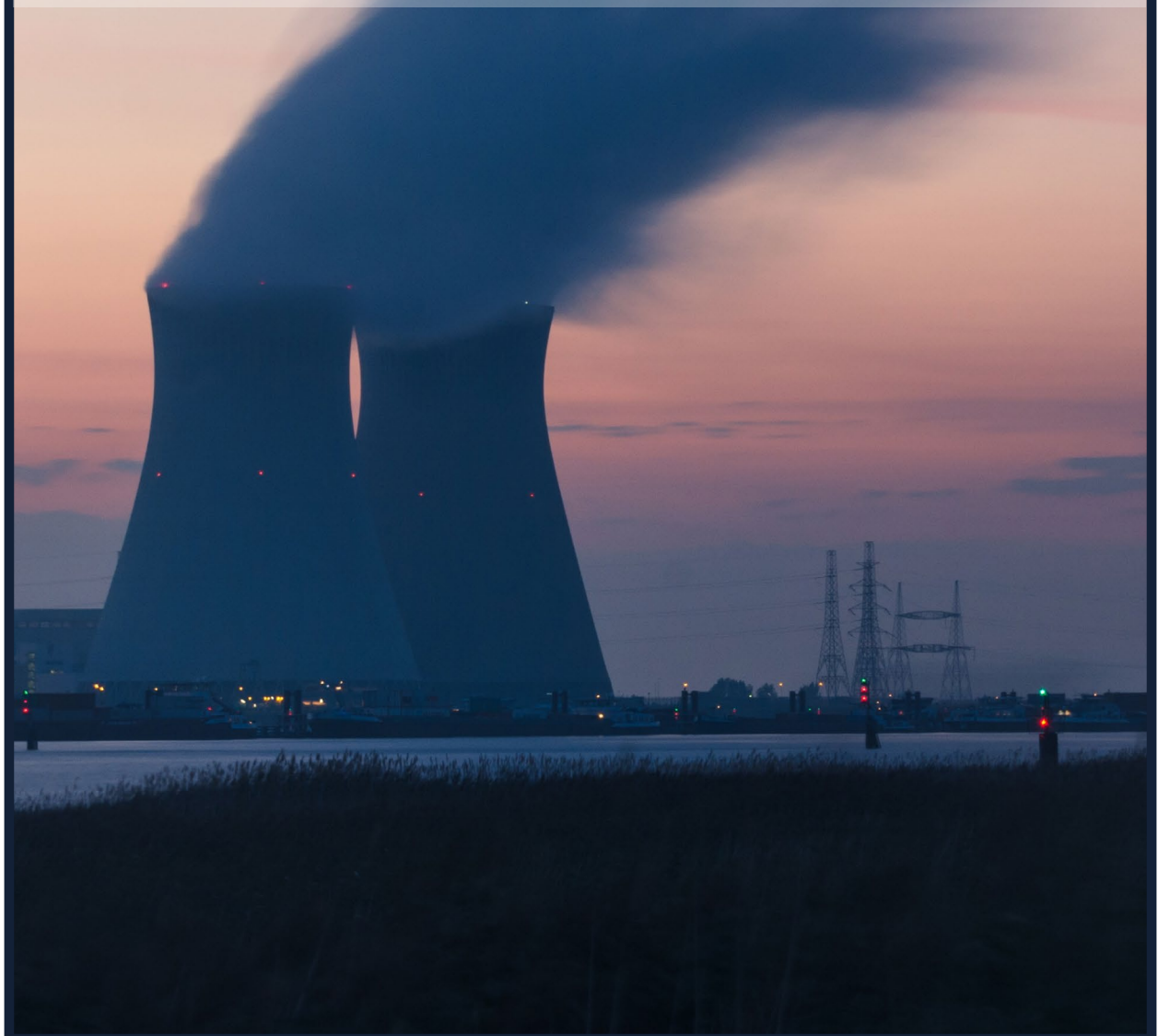
"Nuclear plant cooling tower blowing smoke", Unspalsh, Frédéric Paulussen, 2018
